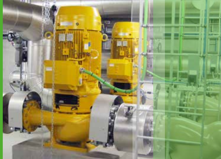
Space saving installation with vertical NSL pumps.
