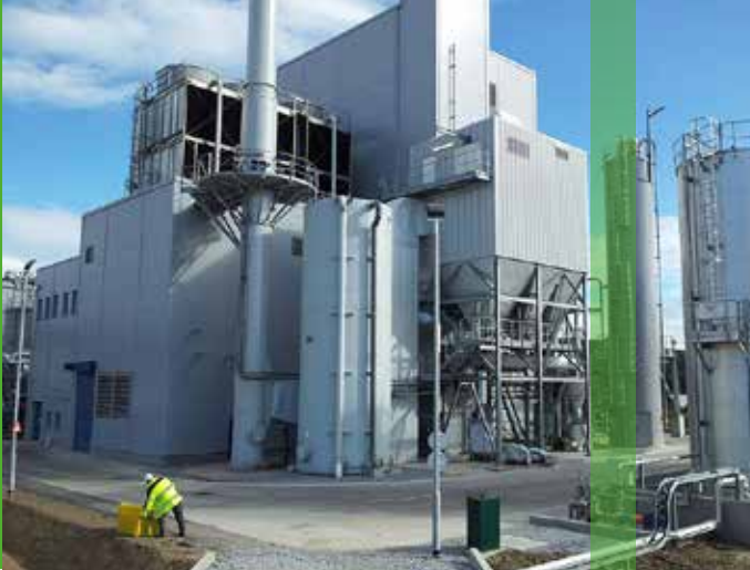
The Helius CoRDe Ltd Plant, Scotland.
